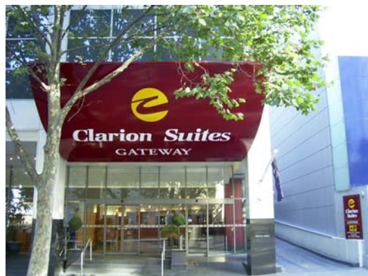
Hotel Entry on William Street
